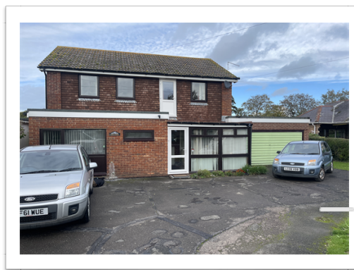
Pic b) 1 The Existing House Front View
